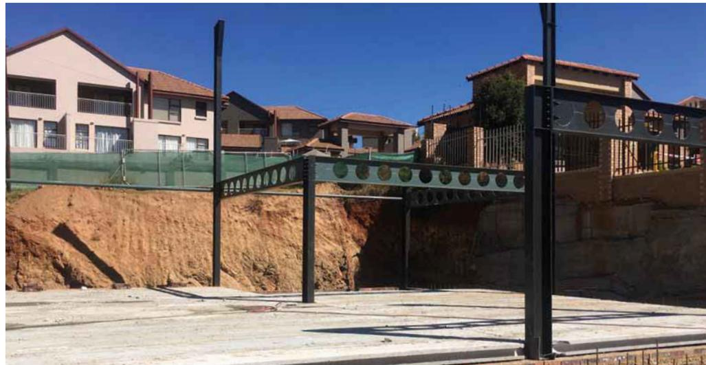
once the steel frame was erected. This created an added benefit of creating a working platform for the construction workers.
