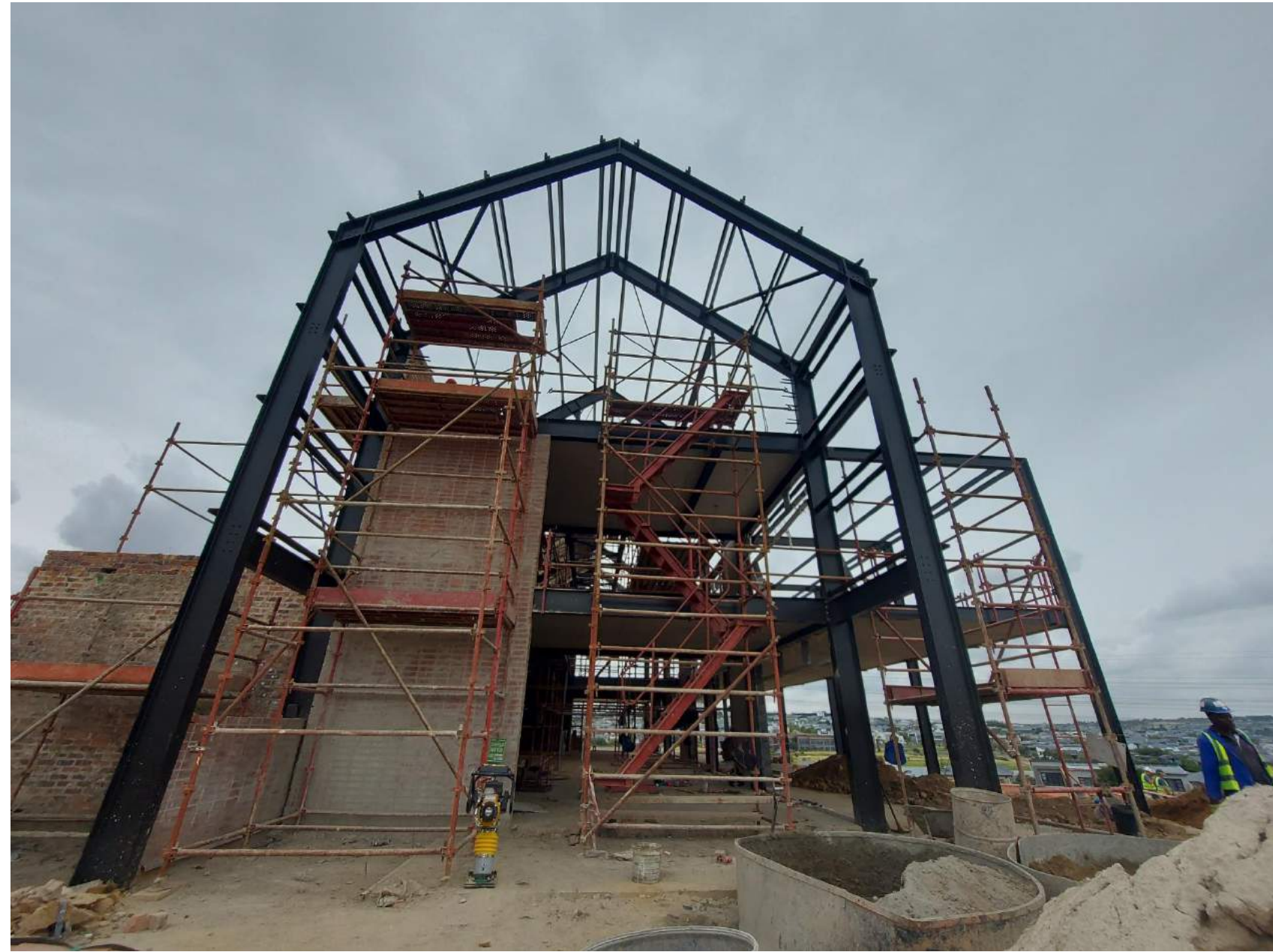
Restaurant is starting to take shape
