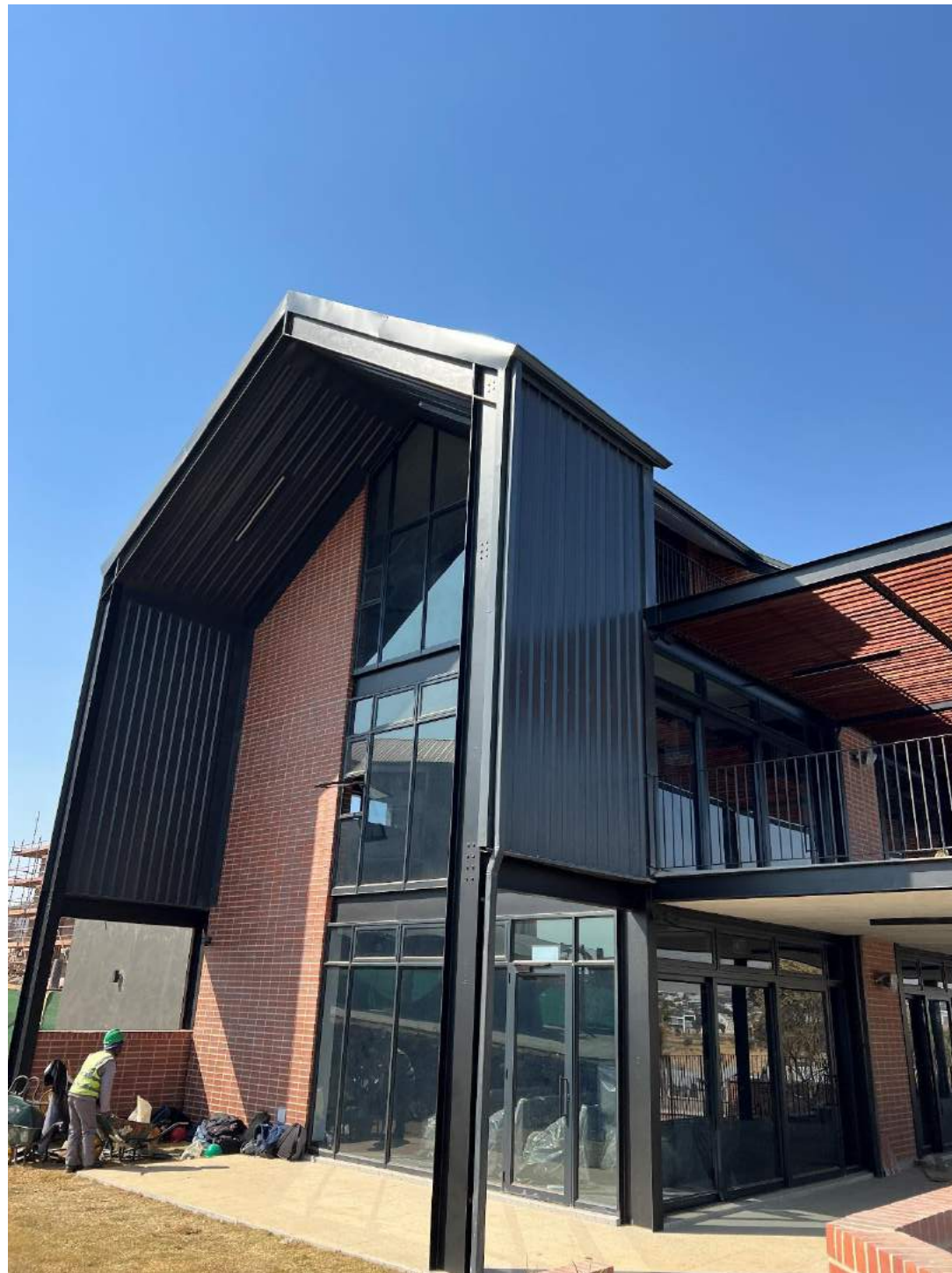
Saffal Coil Rolled into Safintra Widedek
