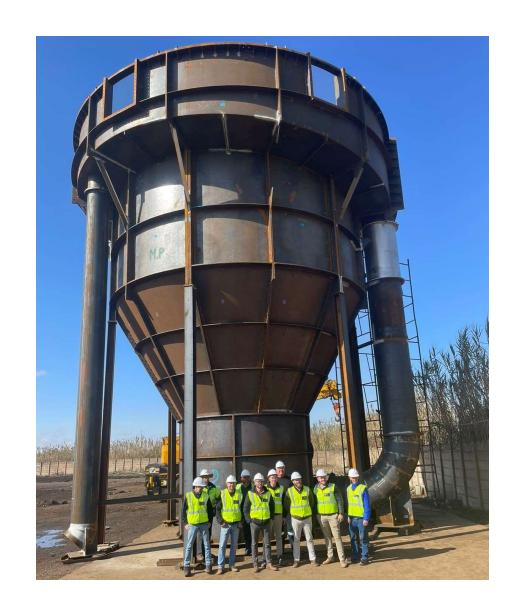
Rubber lining is continuous on the bolted faces. This required that the shop details incorporated the lining thickness and during fabrication that spacer plates were inserted in the connections to simulate the lining.
