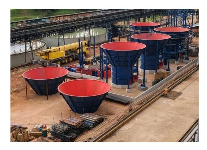
The Reactors were first erected before the adjacent Plant Building could be built over the Reactor laydown area.
