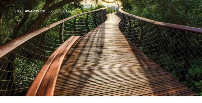
experienced minimum interference from the structure. The surveyor was required to accurately set out the position of each column, and the position and orientation of the two abutments on site, so that when steel was delivered to site, everything fitted.
