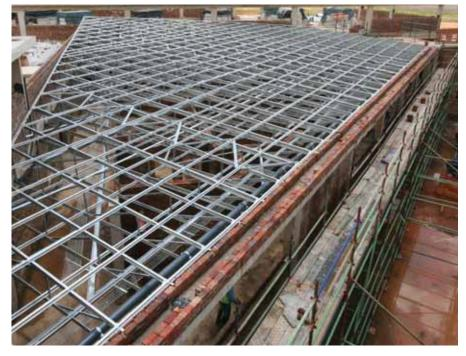
It is a pity that the patients can't appreciate the light steel roof structure of the Mediclinic Midstream in Centurion. Nevertheless the story is an excellent advertisement for light steel frame roofing.
