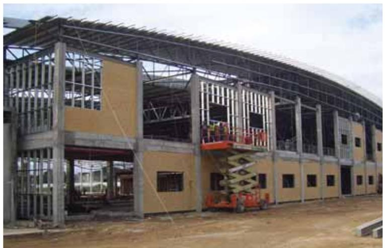
Light Frame Homes (Cape Town) supplied and cladded the light steel frames of the Novo warehouse.
