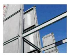
Figure 3: Steel plate shear wall.
