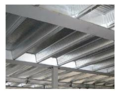
Figure 4: Steel composite slab.
