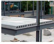
Figure 1: Hollowcore plank on steel.
