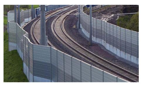
The advanced absorptive materials found in high-performance absorptive noise barriers makes it possible to better mitigate unwanted noise created by rail and aircraft.
