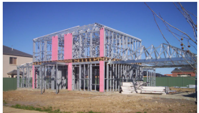
A light steel frame house under construction.
