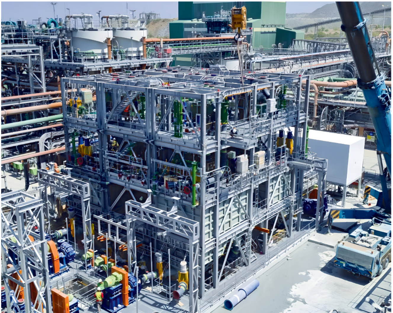
LYCOPodium MODULAR PLANT. Winner of the Mining category at the Steel Awards 2025.
